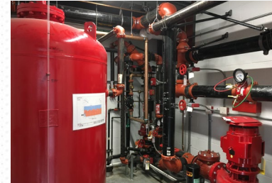
Cleaning of fire-fighting systems
